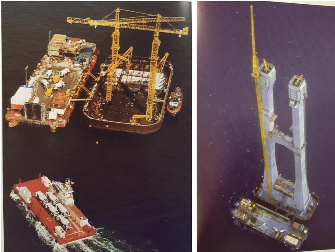
Figure 6. Pictures of construction/working pontoon for construction of East bridge pylon Storebælt. ("Concrete Technology, The Storebælt Publications, 1999")
